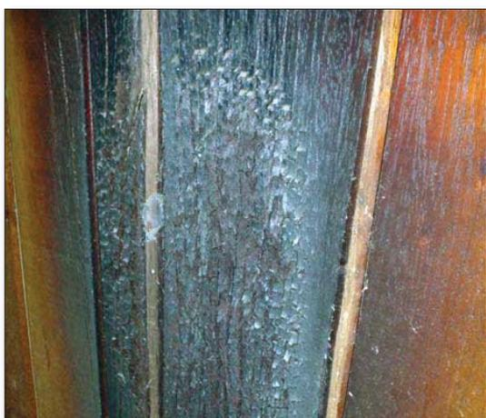
Burned timber panel on casing
