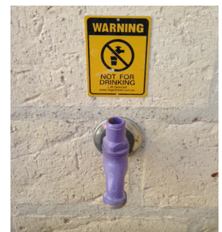
Image 1: non-drinking (recycled) water signage and tap
