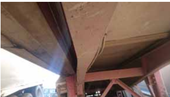
Damaged longitudinal structural element
